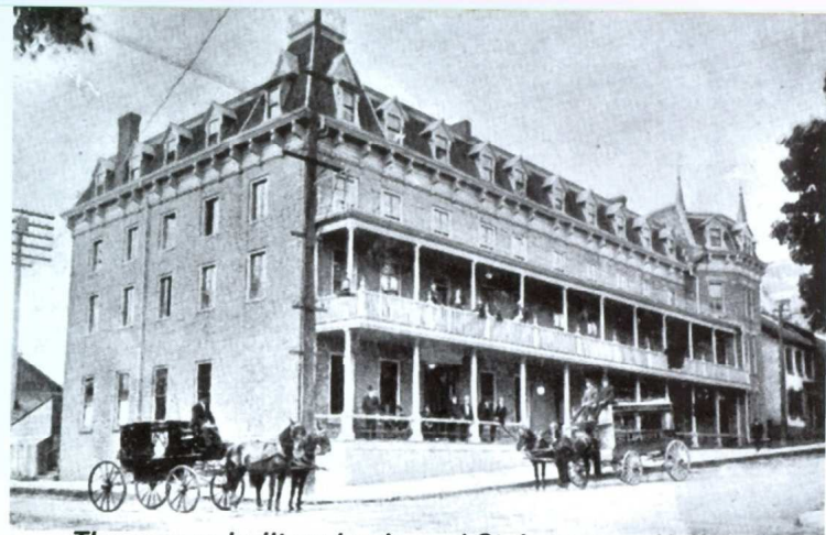
The new re-built and enlarged St. Lawrence Hall as it appeared about 1895, following the disastrous fire of 1883.
