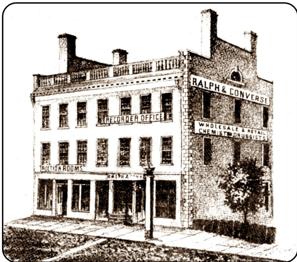
The earliest picture of the Jones-Harding Building is this engraving based on a daguerreotype taken in 1852.
